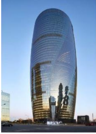
Leeza Soho Tower Tasarımcı: Zaha Hadid Architects Yer: Pekin
