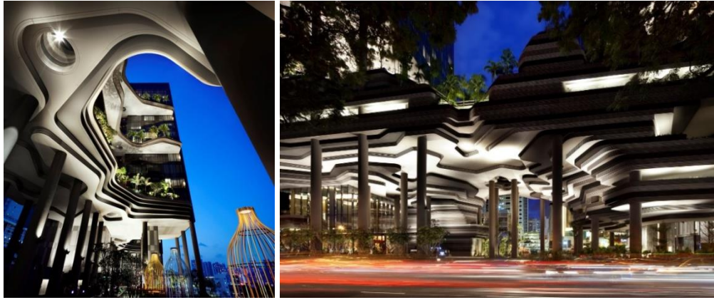
Resim 77. Otel ParkRoyal Collection Pickering Cephesi, Singapore (URL-46)
