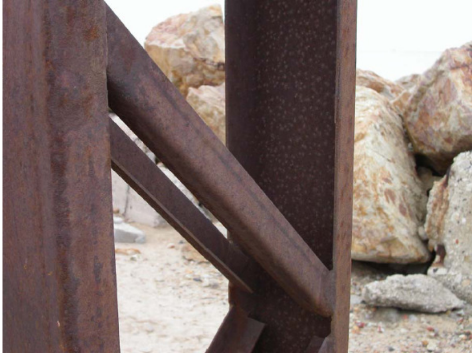
Figure 3.18: Welded areas with no significant corrosion (NN 2007).
