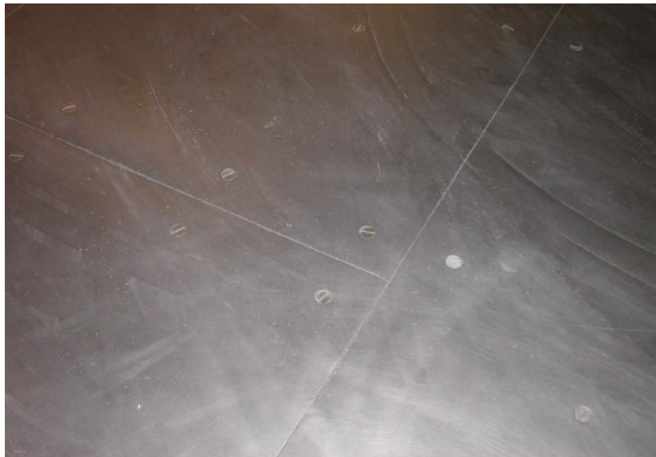
Figure 3.16: 6 x 1000 x 200mm 3Cr12 plates bolted to the dodgem car floor (NN 2007).
