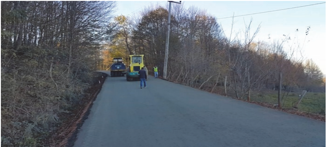
Şekil C.11. Son silindiraj (mix-type compaction)
