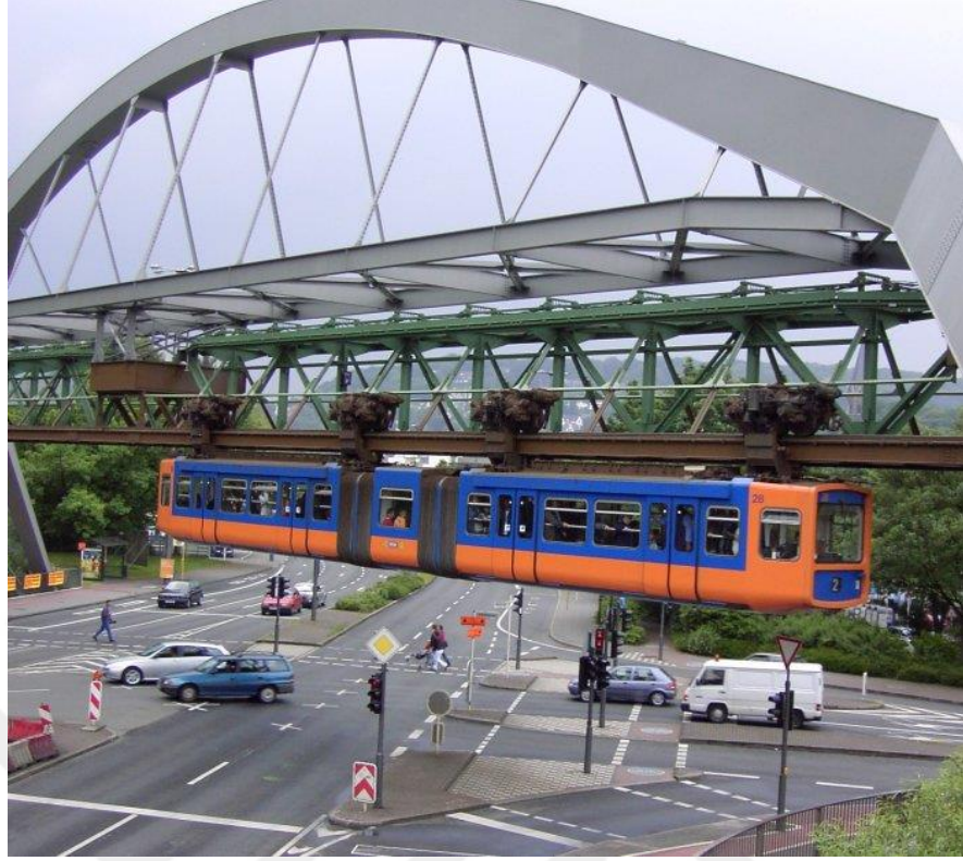
Şekil 1.7. “Wuppertal Suspension Railway” [29]
