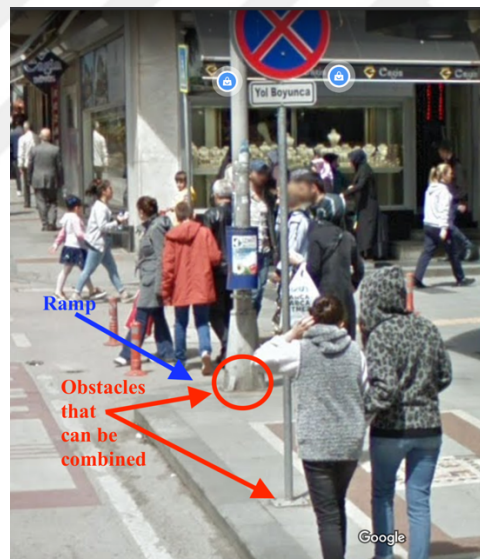
Figure 2.1. An example of an obstructed ramp (URL-23)
